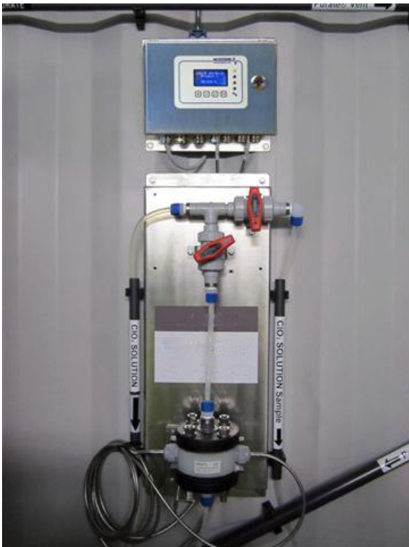
Kemtrak DCP007 process photometer ClO 2 installation
